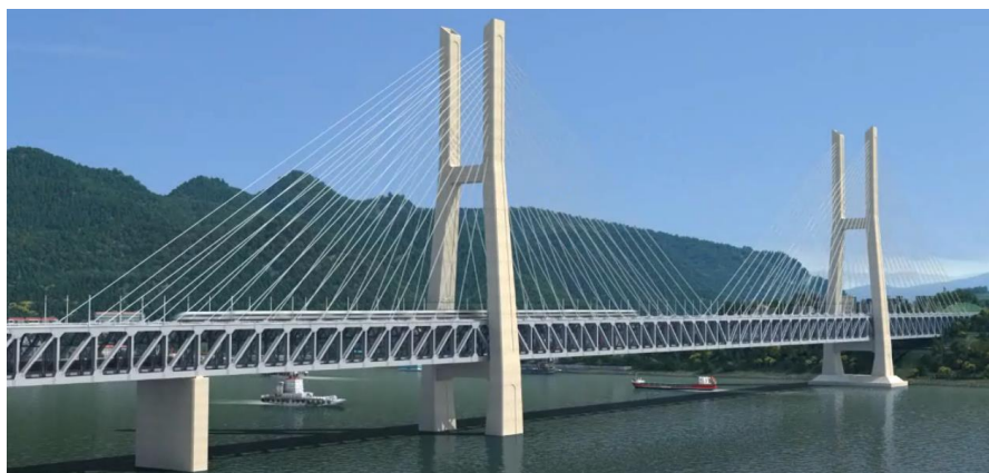
Fig. 4: The new Baishatuo Yangtze River Bridge
